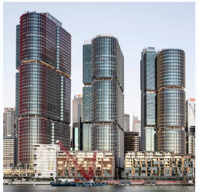
Barangaroo South Precinct / Source: Lendlease
